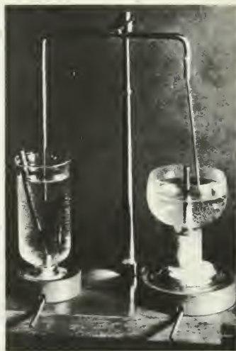
Two versions of Faraday's electromagnetic rotator. In each, the cup was filled with mercury so that a large current can be passed between the base and overhead support.
