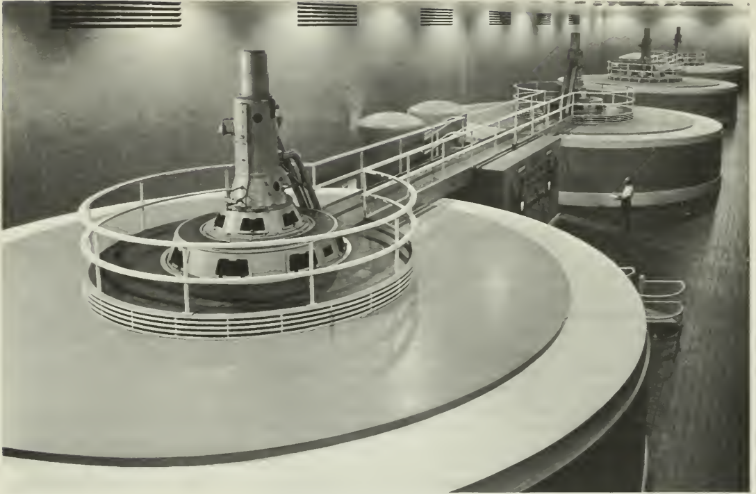
Water-driven electric generators producing power at the Tennessee Valley Authority. The plant can generate electric energy at a rate of over 100,000,000 watts.
