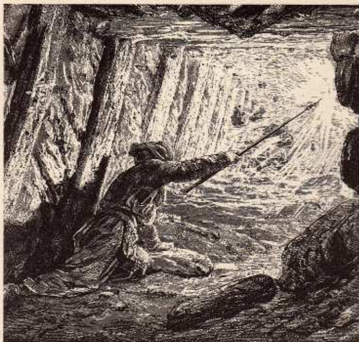
Before proper ventilation was introduced, the 'penitent' (or fireman) got rid of the gas in the mines by igniting it. His job, as you may imagine, was not a popular one.
