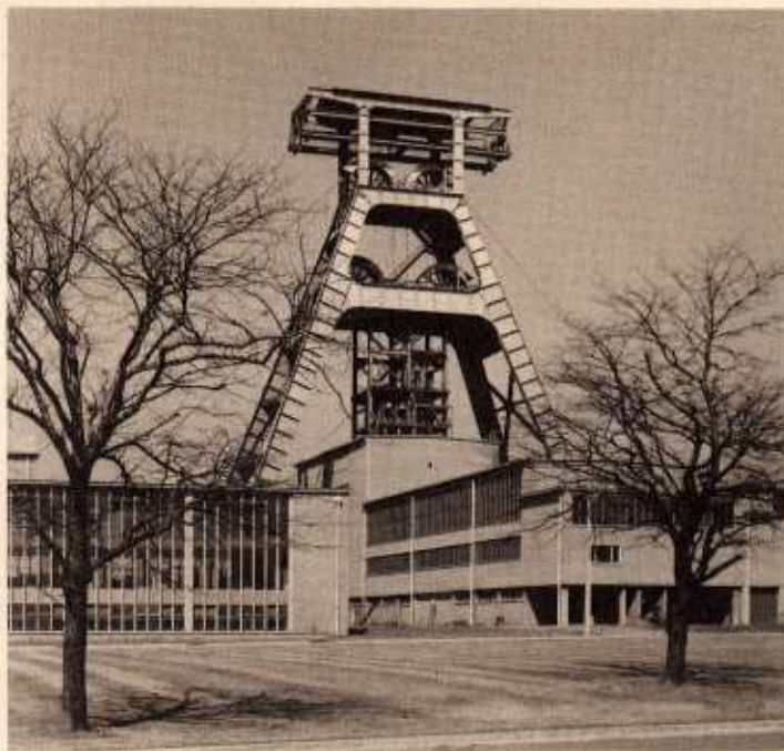
above At the surface of an up-to-date mine — Hem Heath Colliery, near Stoke-on-Trent. Apart from the pithead winding gear, above the access shaft to the coal seams, it looks like a well-laid-out factory.
