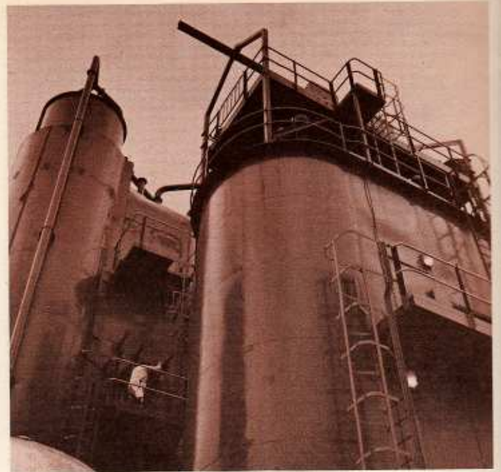
Liquid air is separated into its different chemicals in this huge distillation column. British Oxygen Co.
