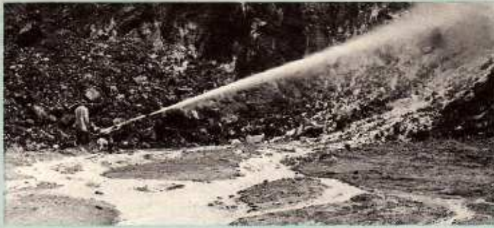
Washing china clay (kaolin) from the pit face with a high-pressure hose. English China Clays Group
