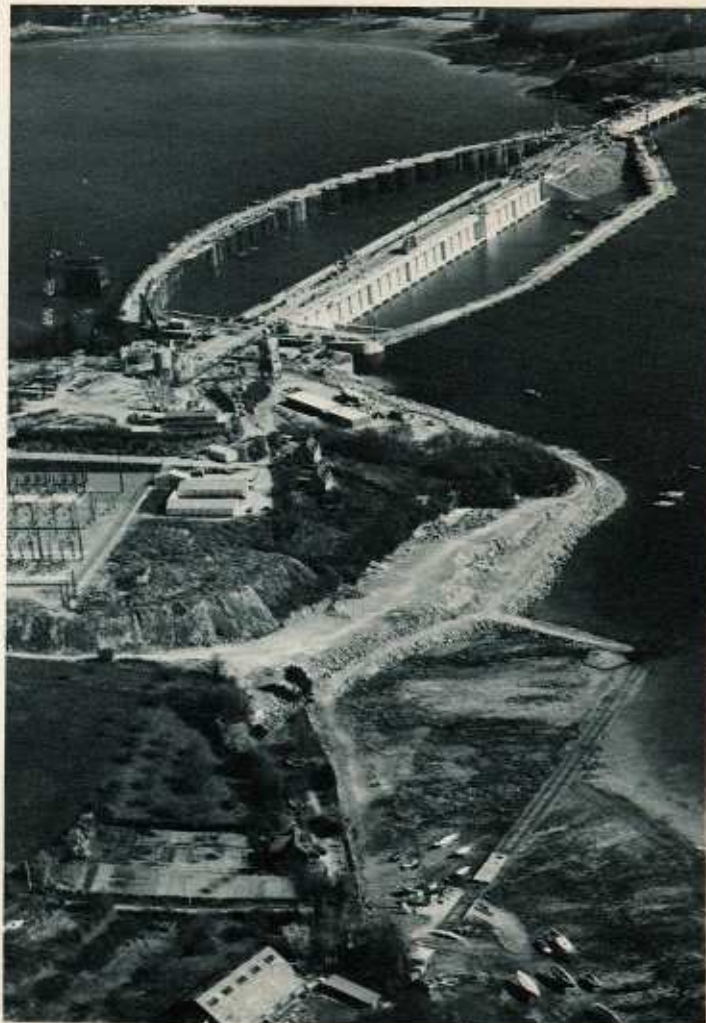
The tidal power station in the Rance estuary. Water drives the turbines in the semicircle of cylindrical drums as the tide rises and as it falls again. French Government Tourist Office
